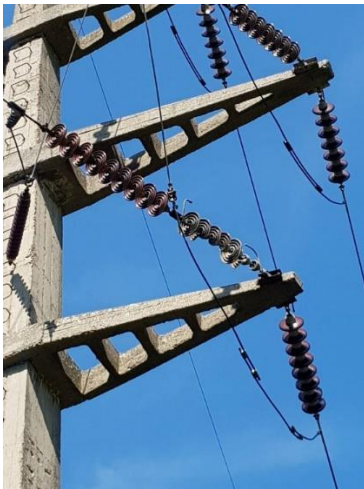
Figure 10: Damaged insulator.
