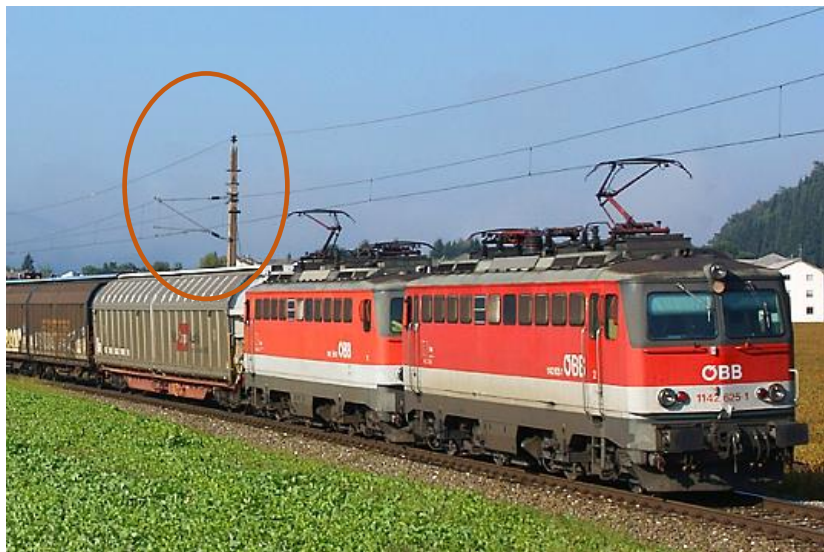
Figure 2: Railway overhead track in the analyzed section; Tower structure highlighted; © Markus Hipfl, bahnbilder.warumdenn.net
