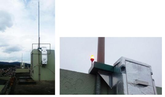
Figure 5. Current sensor installed on the lightning rods (left) and detail of the installation (right).
