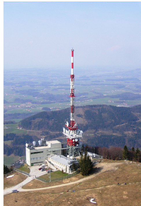
Fig. 1. Radio tower at Gaisberg with nearby operational buildings
